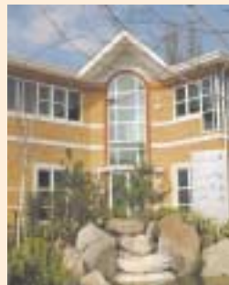
One of the pre-let offices
